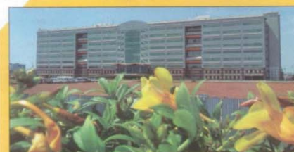
▲ The Chennai One IT Park is amongst the world's largest Gold Rated Green buildings under the LEED Green Building Rating System.
